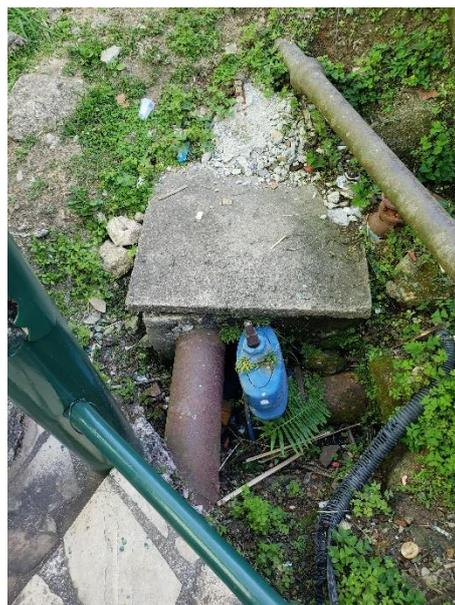
FIGURA 246 – EXTRAVASSOR DO RESERVATÓRIO
