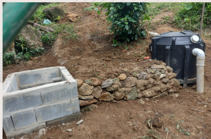
Biodigestor instalado
